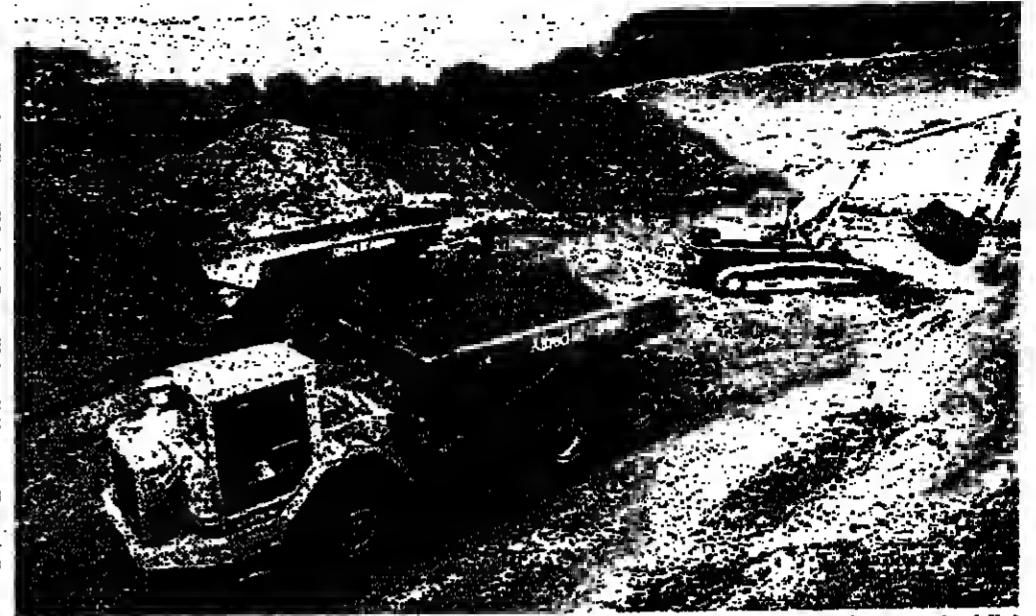
Work on the Greatford-Pufford By-pass, on the Welsh border near Wrexham, part of an eventual link between Chester and the M54
